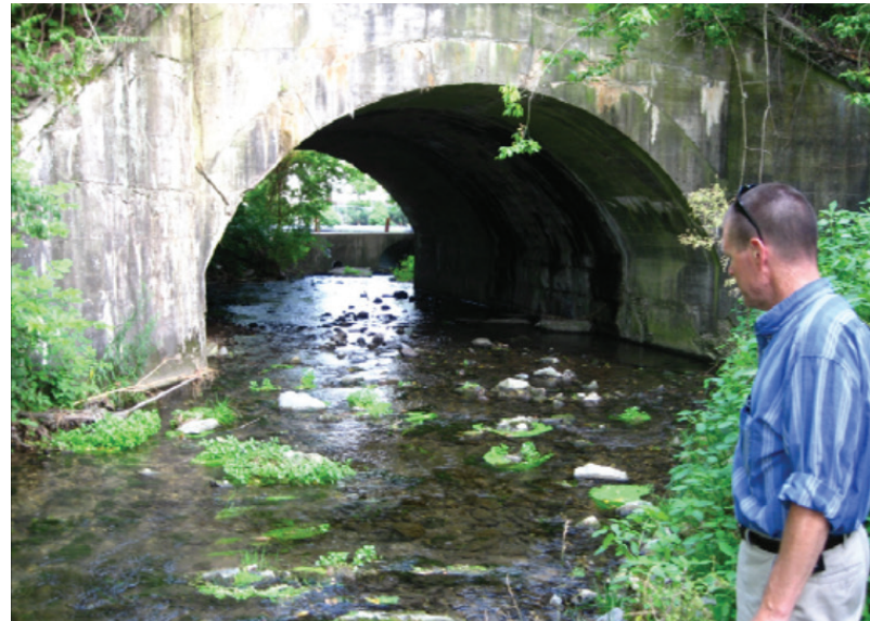
2. Location for potential pedestrian tunnel at existing culvert
