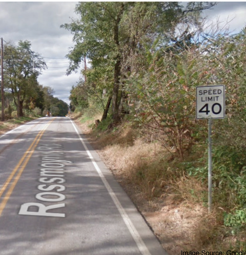
Existing Conditions: Rossmoyne Road
