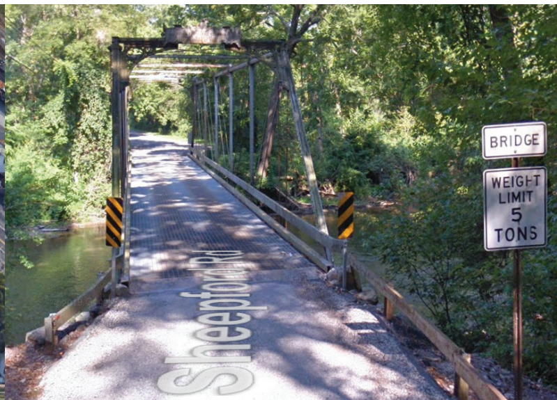
Existing Conditions: Bridge at Sheepford Road
