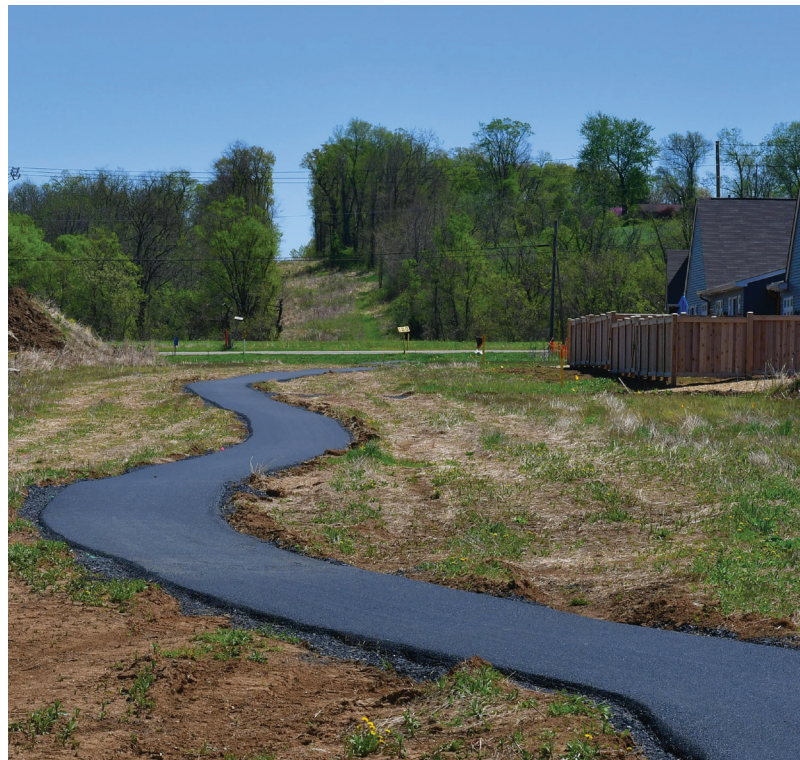
Trails Under Construction at Arcona Development
