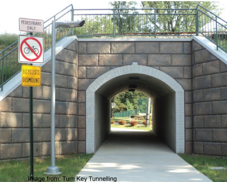
Image from: Turn Key Tunnelling Potential Solution
