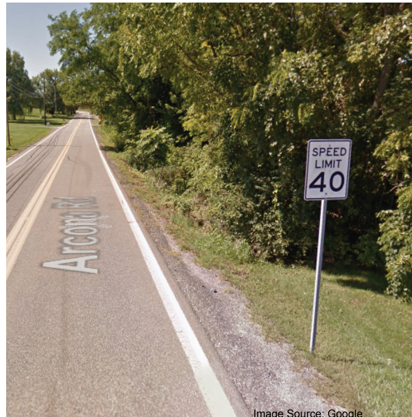
Existing Conditions: Arcona Road
